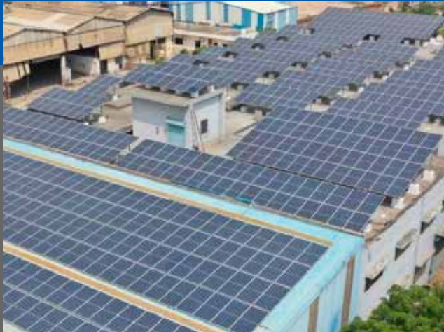
700 kWp Lucknow, Uttar Pradesh
